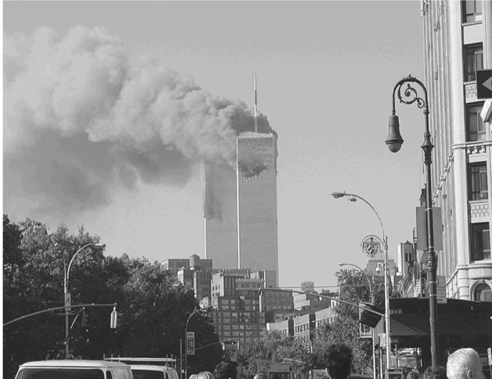
FIGURE 1.1 World Trade Center towers on September 11, 2001, at 9:05 a.m., looking south from 6th Avenue and Washington Place, New York, N.Y. (Architect: Minoru Yamasaki with Emory Roth and Sons; photographer: Bruce D. Eisenberg, AIA.)
