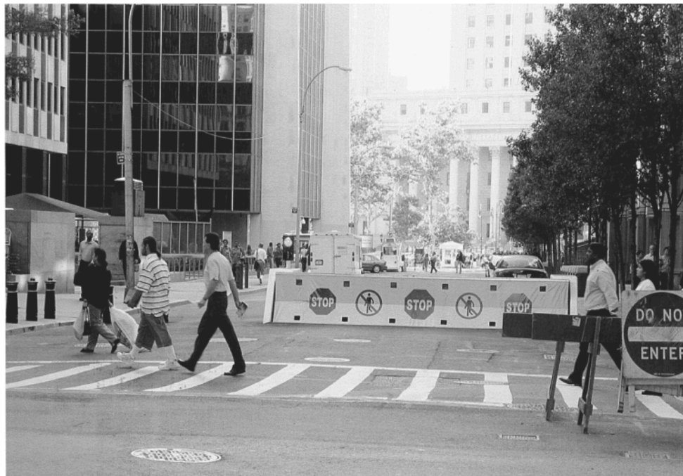
FIGURE 1.15 Concrete barrier limits vehicles at Federal Plaza, Duane Street, Lower Manhattan, New York. (Photographer: Mark Ginsberg, AIA.)
